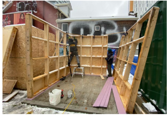
Figure 4: Construction of Test Hut (Johns, 2023)
